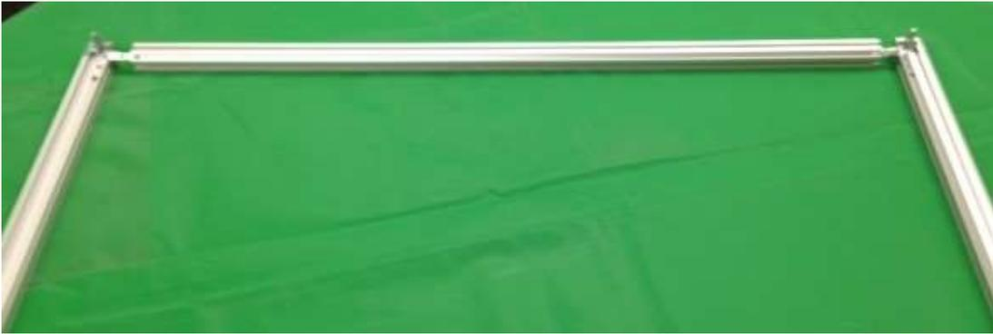
7. Place Plexiglas side into the groove of the assembly and attach the fourth 29" aluminum tube, making a square assembly. (Side Assembly)
